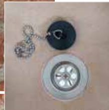
Mesh drain with plug
